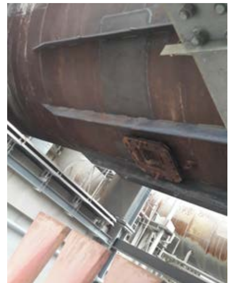
Kiln crack repair
